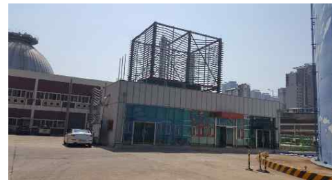
Biogas-to-Vehicle Fuel Project at Sewage Treatment Plant in Busan
