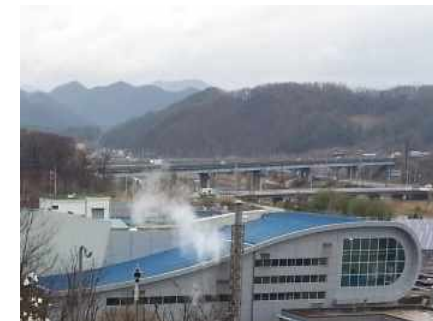
Sewage treatment plant fuel supply (Approx. 1,500 Nm 3 /d)
