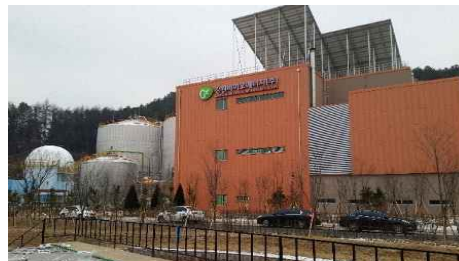
Wonju Organic Waste Biogas Plant
